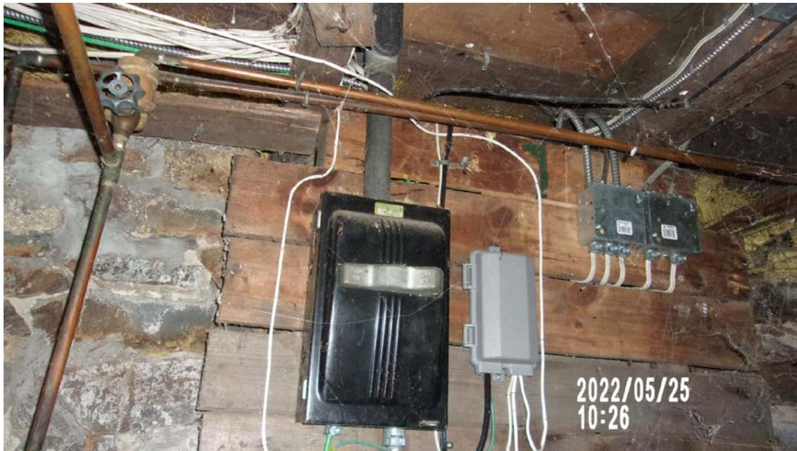
E3- Amalgamated Main Fusible Disconnect Switch Fused at 60 Amps.
