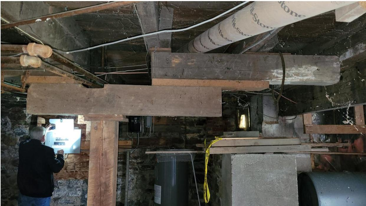
This section of floor should be temporarily reinforced as soon as possible. A couple of jack posts will stabilize this area. The foundations walls for the original building are constructed with stone and they are generally in good condition. There is a crack in the foundation wall between the original building and the East addition and this should be repaired at some point. See the photograph on the following page.
