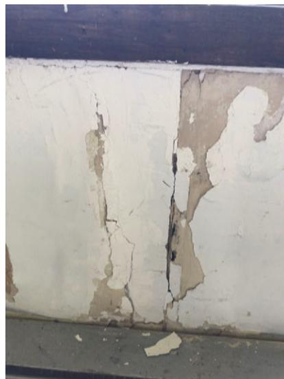
*Water damaged drywall underneath sliding window*
