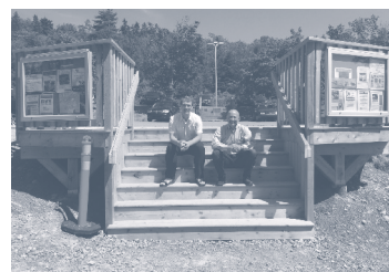
New stairs at Shubie Park.
