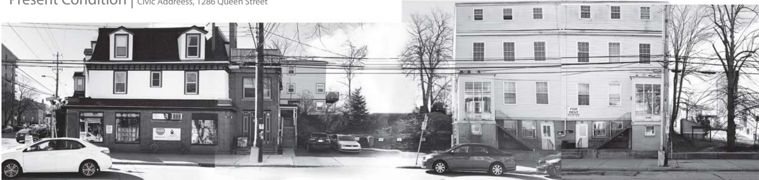
Present Condition | Civic Address, 1286 Queen Street
